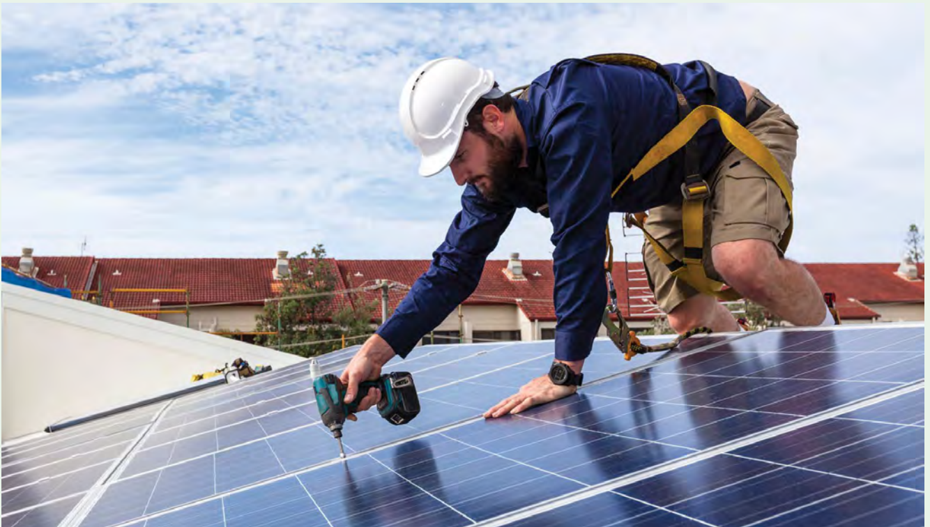
Solar panel technician
